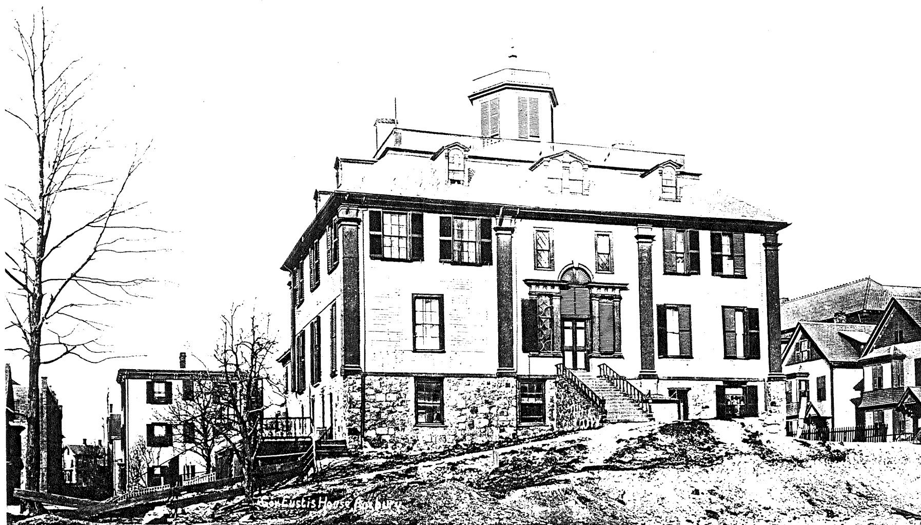
Fig. C-4. "Gov. Eustis House, Roxbury", photo from east, 1890 by W. F. McIntire. Earliest photo of east front before construction of adjoining buildings showing surviving piazza base, double dormer and twin second floor sash added. (SPNEA Neg.)
