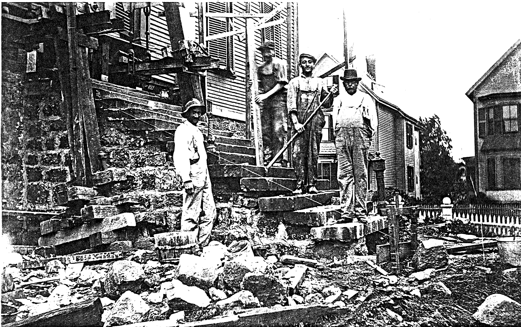
Fig. C-11. Shirley-Eustis House, southeast view of east front steps and workmen, "Mr. Bowen," contractor, during 1915 repairs. Photo by Lillie B. Titus, Shirley-Eustis House Association. (SPNEA Neg. 6636-B)
